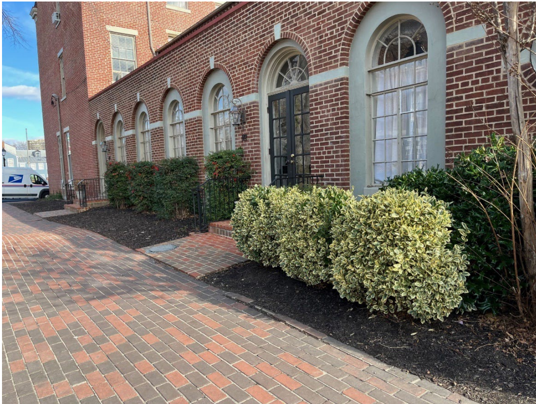
Figure 1: West elevation showing narrow "yard."
