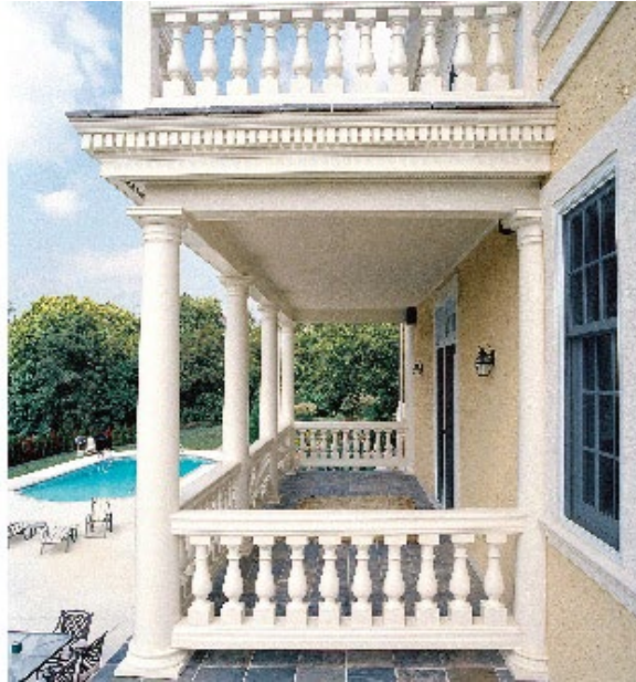
Figure 6: Fypon Classic baluster installed
