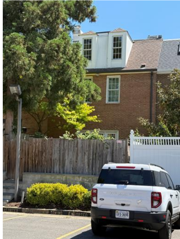
Figure 7 - Rear View from the Parking Lot
