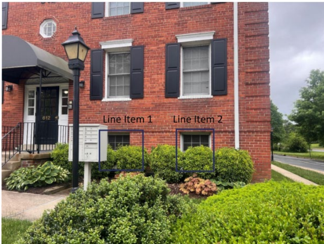
Figure 1 - Windows to be replaced
