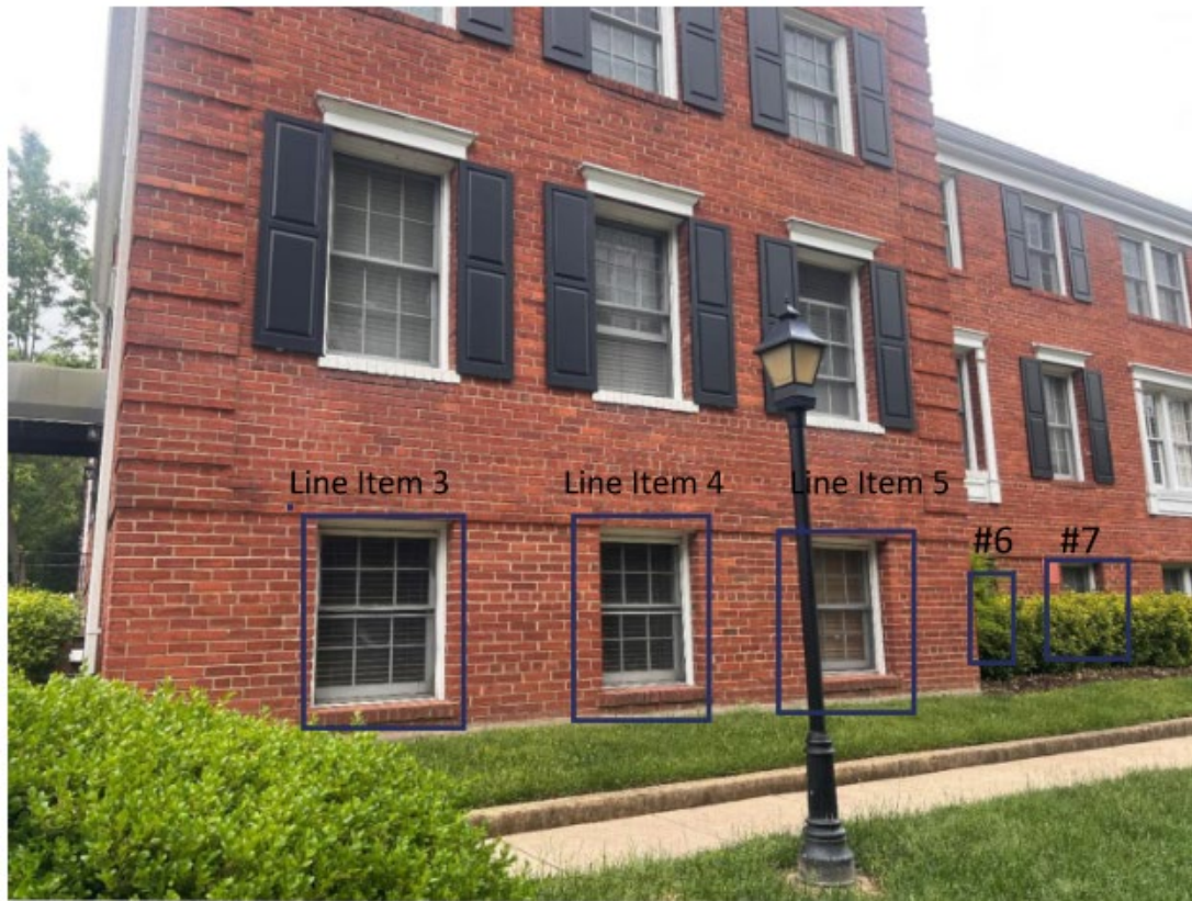
Figure 2 - Windows to be replaced
