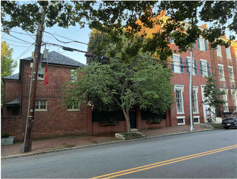
EXISTING FROM (NORTHEAST) ON DUKE STREET
