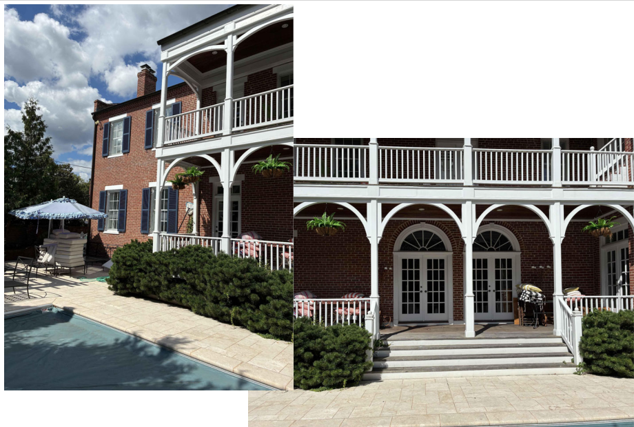
EXISTING PHOTOS AT EXISTING EAST WALL
