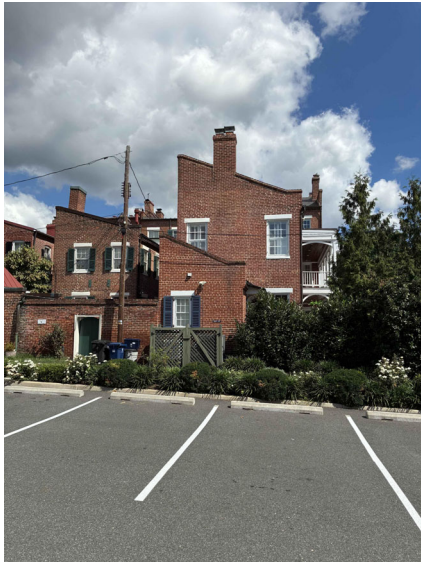
EXISTING FROM (SOUTH) ST. MARY'S PARKING
