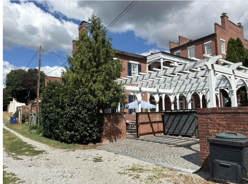
EXISTING FROM (SOUTHEAST) ST. MARY'S PARKING
