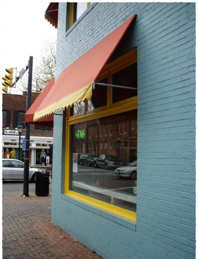
TYPICAL AWNING/WINDOW DETAIL FRAME TO REMAIN-FABRIC TO BE REPLACED (FACING SOUTH-WEST) 801 KING STREET
