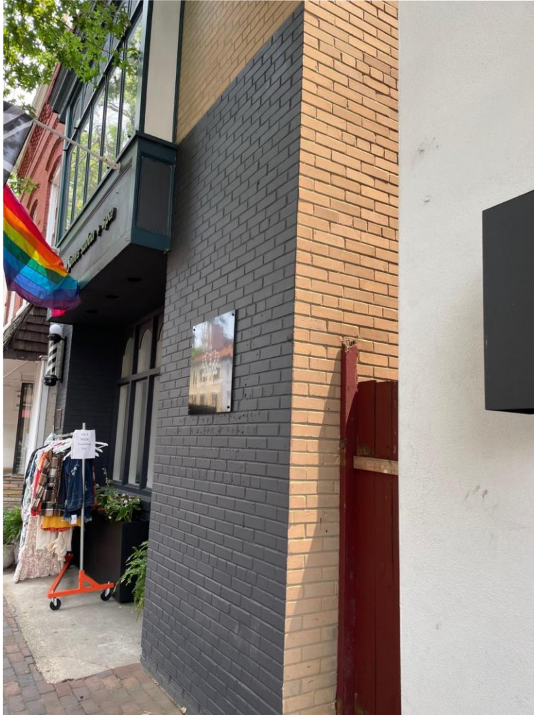
Figure 2 - Painted portion of the building
