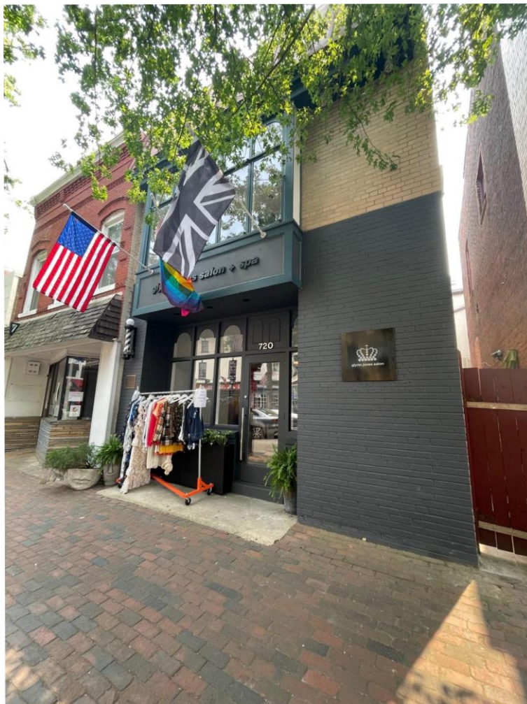
Figure 1- 720 King Street facade.
