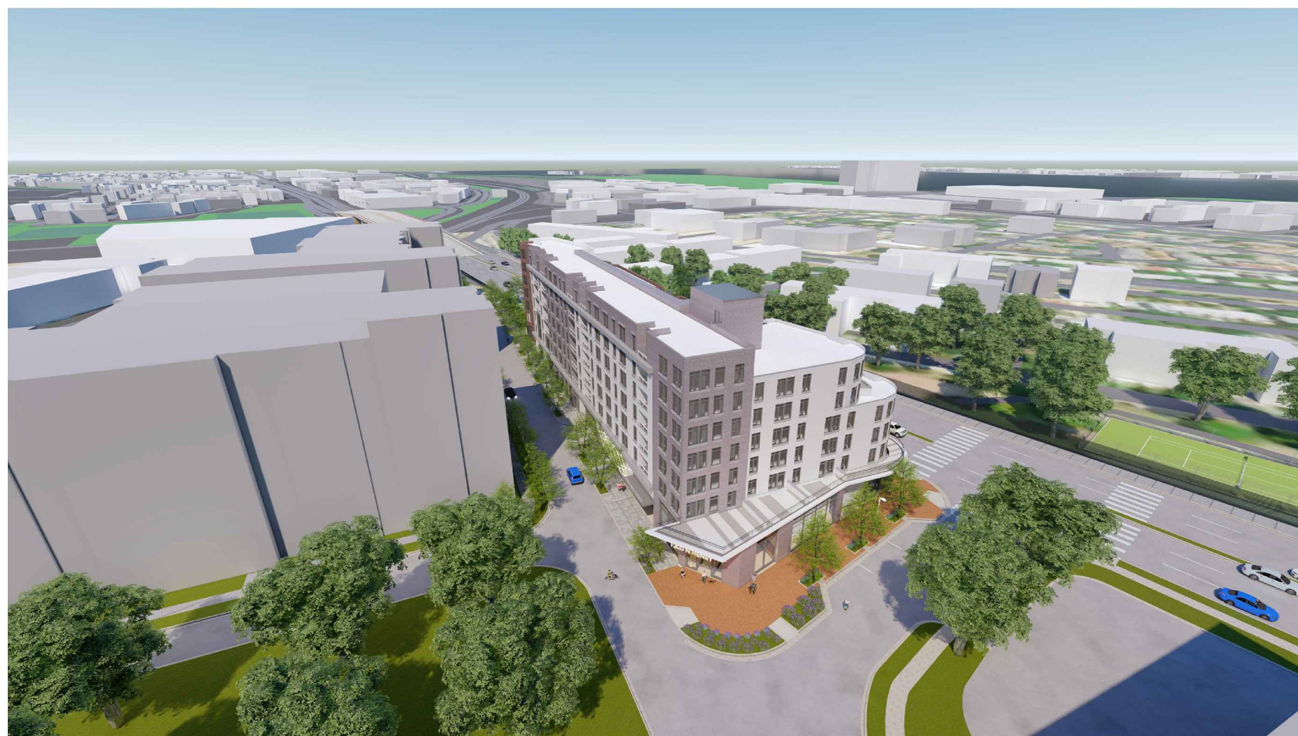
3 SOUTH WEST - AERIAL VIEW
