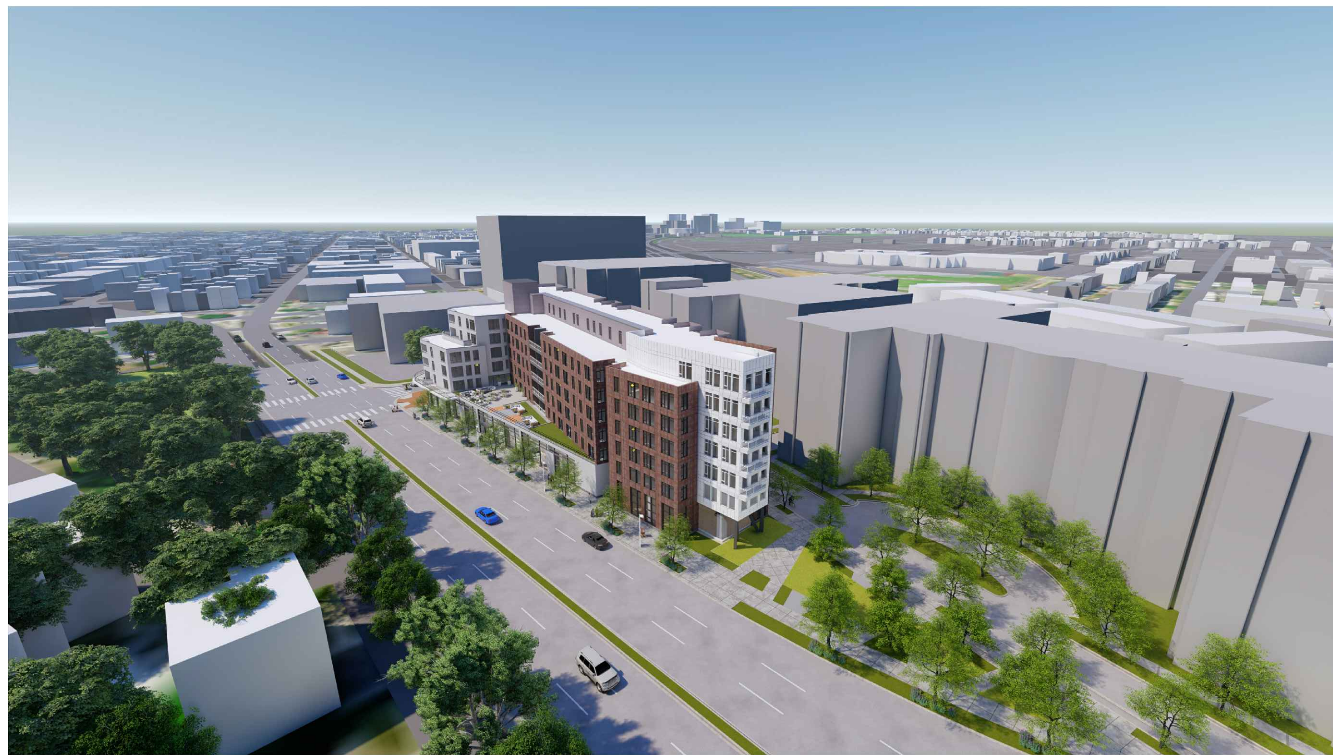
1 NORTH EAST - AERIAL VIEW
