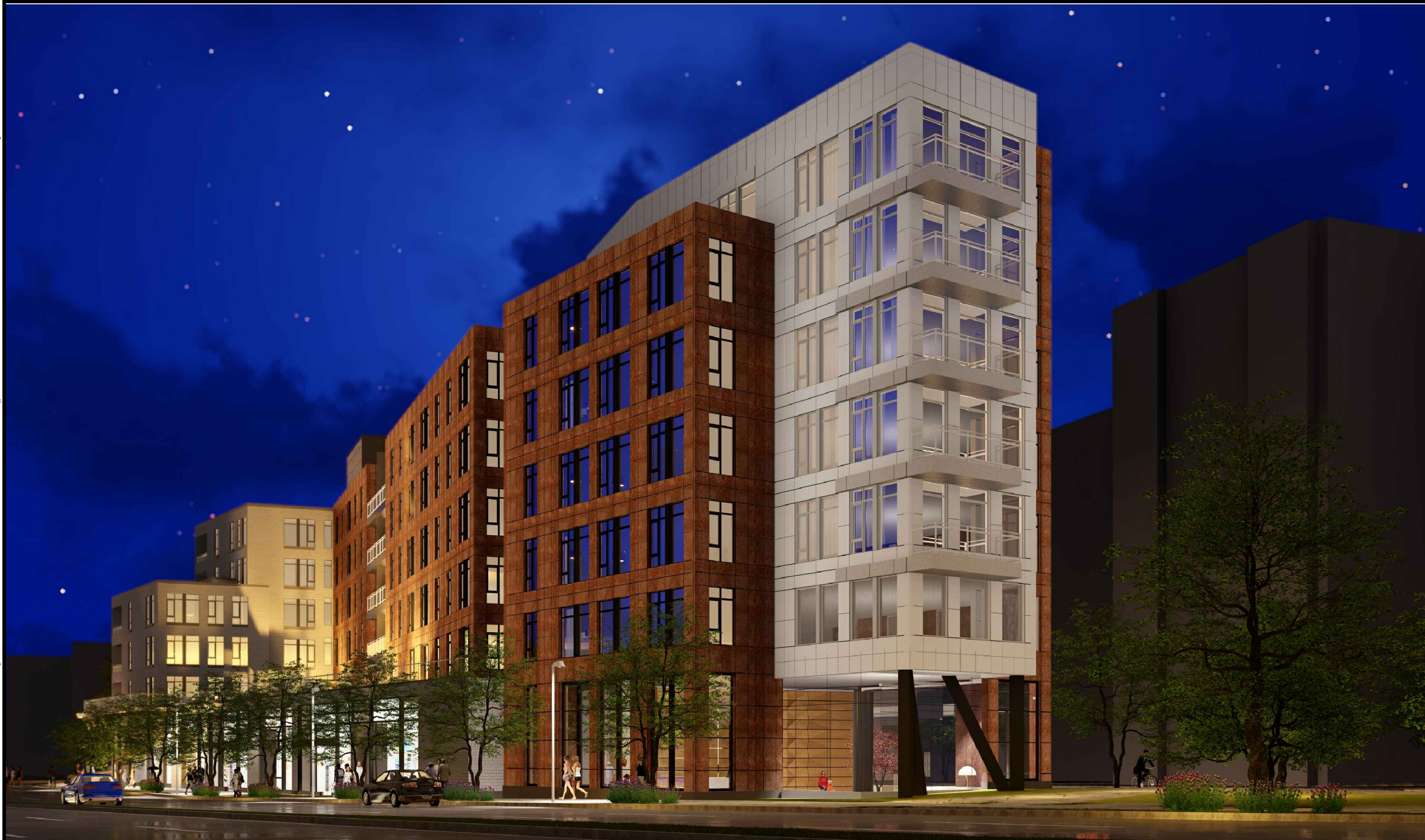
1 NORTH EAST - AERIAL VIEW
