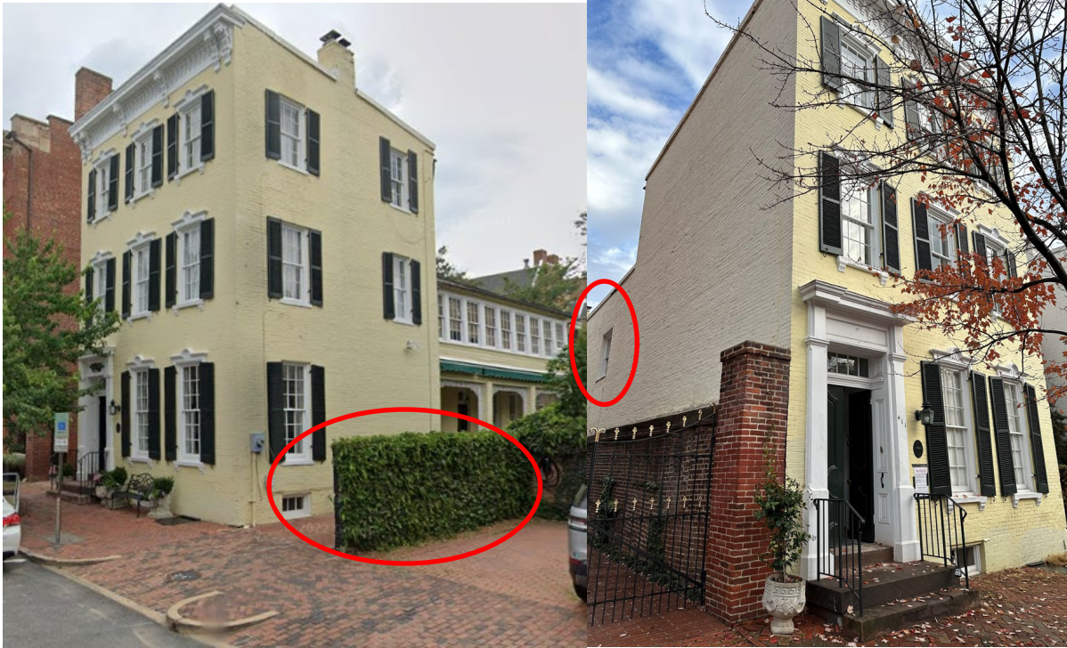
Figure 1: Proposed brick wall to be replaced (left) and window to be infilled (right)
