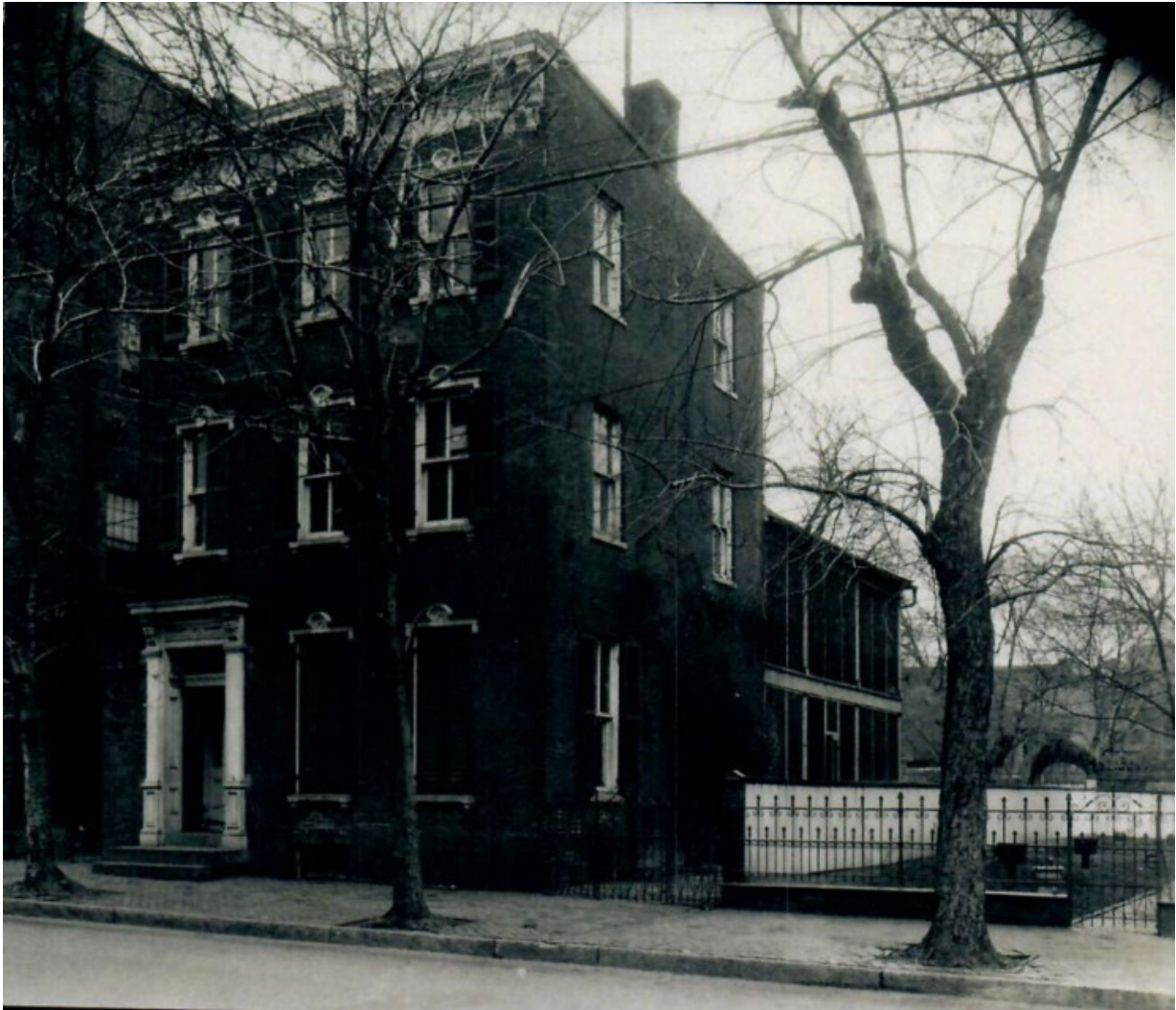
Figure 2: Photograph showing site configuration prior to the construction of the subject brick wall
