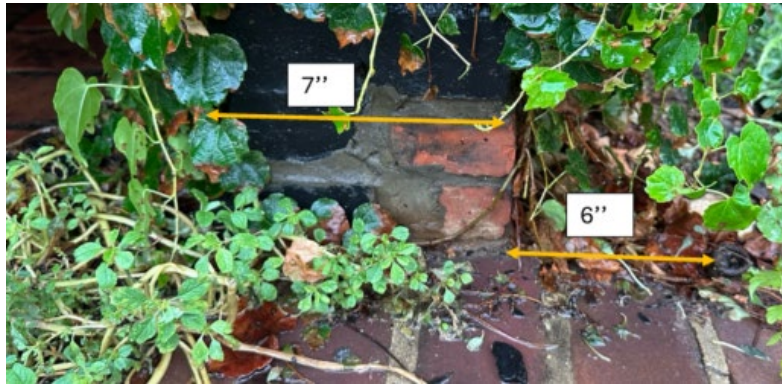
Figure 3: Photograph showing existing fence relative to the property line marker
