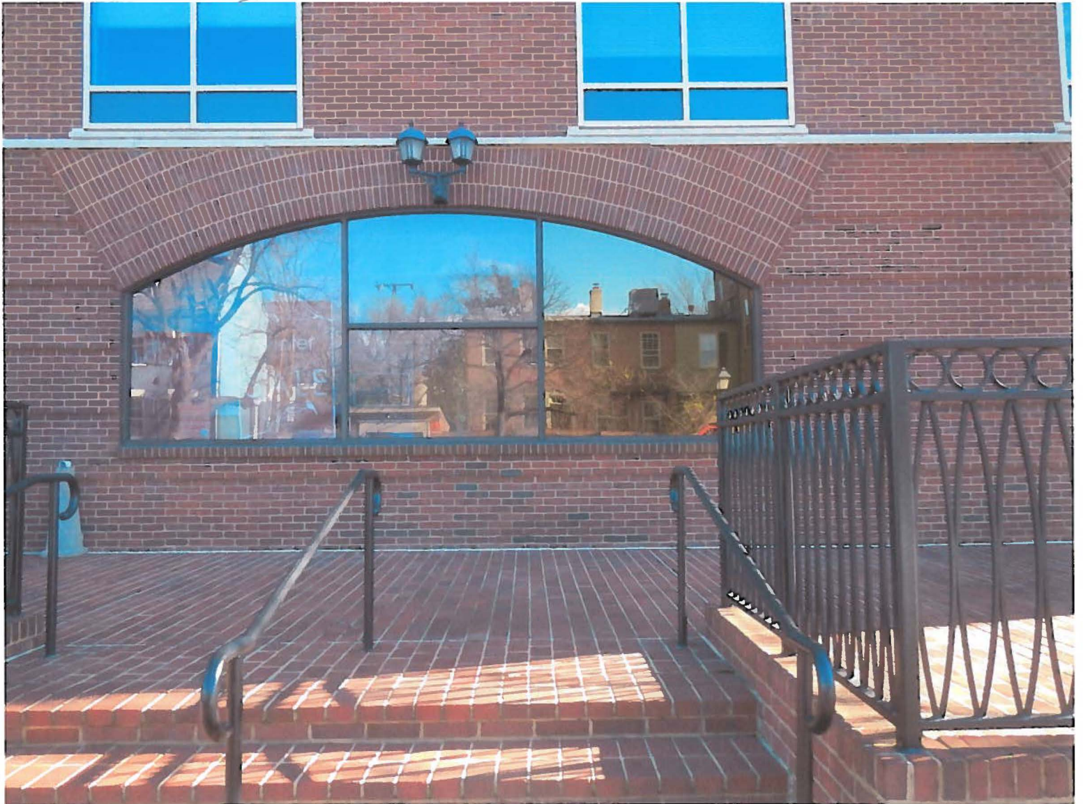
Existing Conditions. Side of Building - S. Columbus St.
