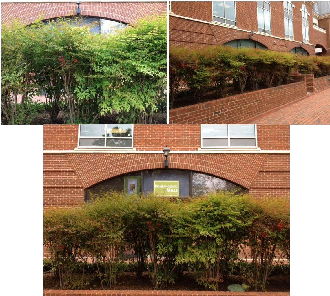
Figure 4-6: View of subject storefront from Duke Street showing obstructive vegetation
