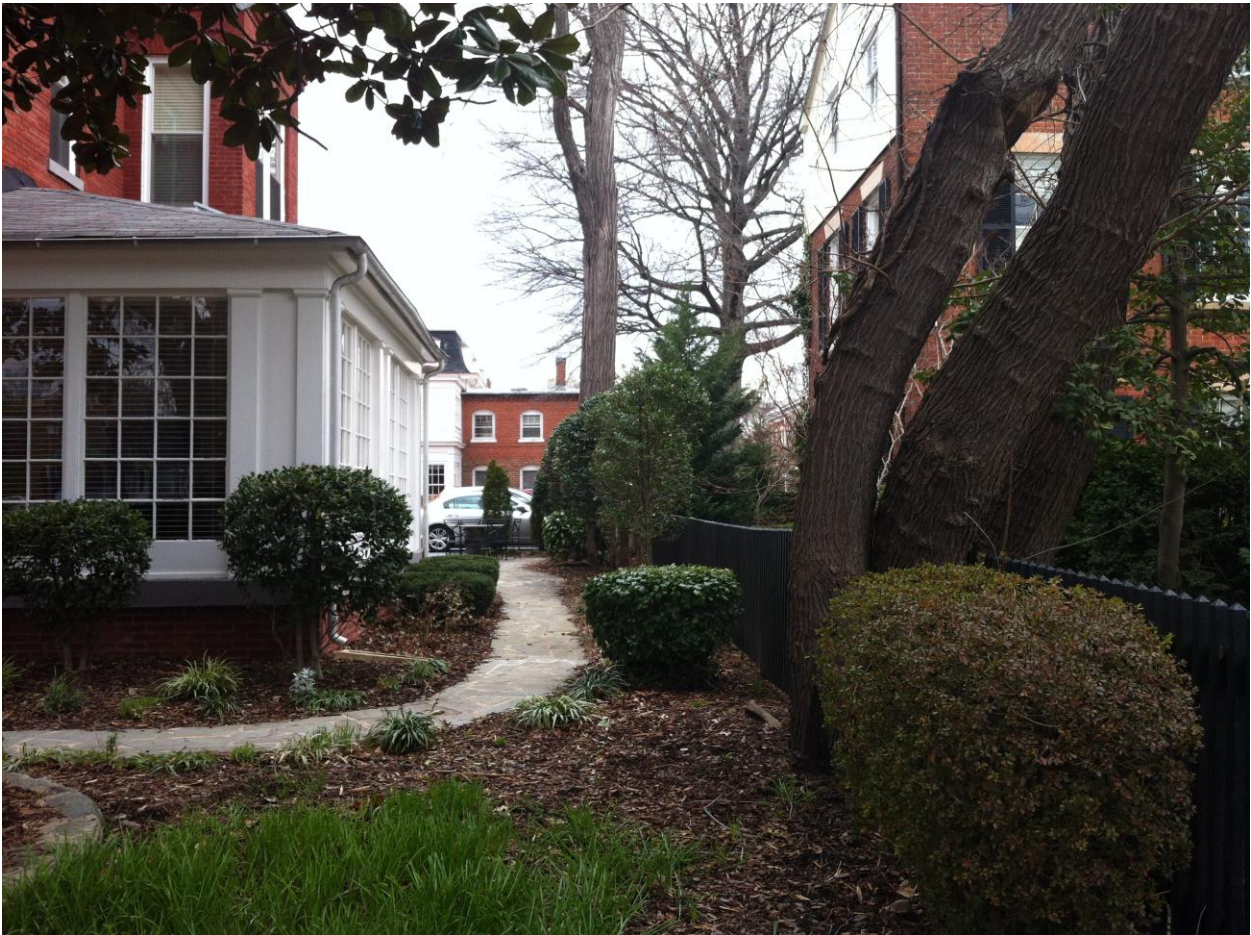
Figure 1 View from Prince Street, looking north. Proposed changes to the rear porch are behind the bushes beyond.
