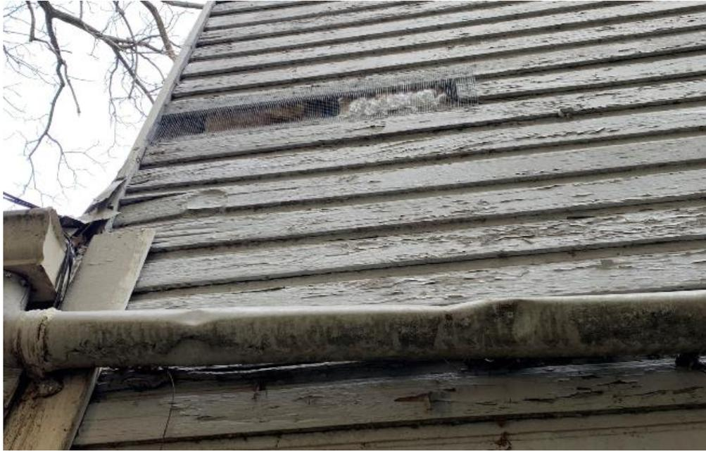
**Figure 2: View of opening in siding at south elevation**
