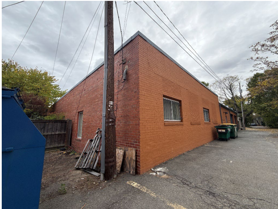
Figure 5: Overview from Parking Lot – East Elevation View to the West
