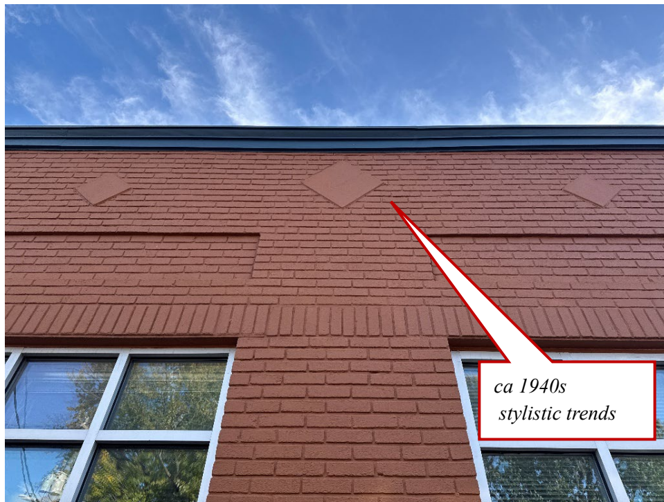
Figure 10: Detail of Parapet – West Elevation View to the East
