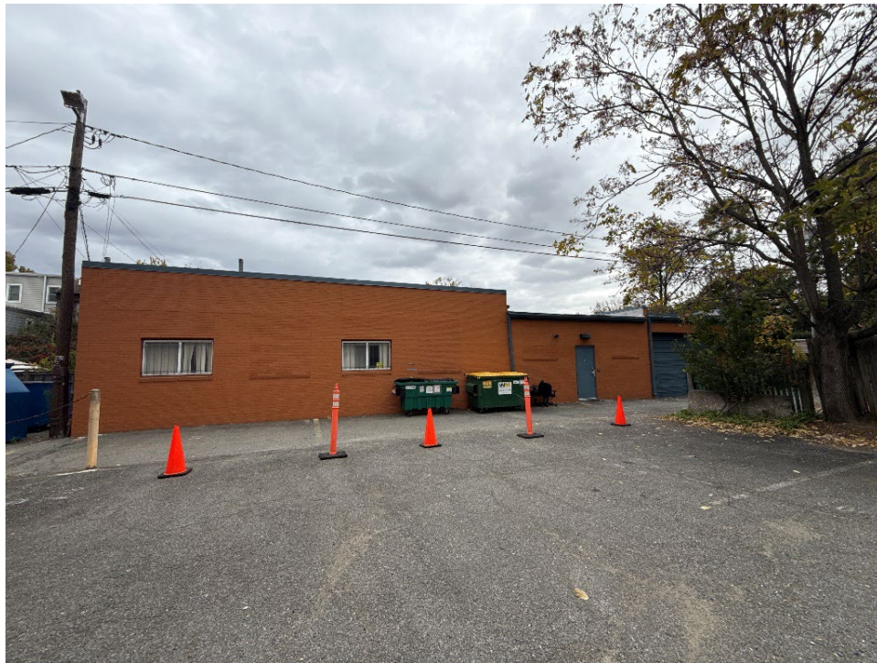
Figure 4: Oblique – South and East Elevation View to the Northwest
