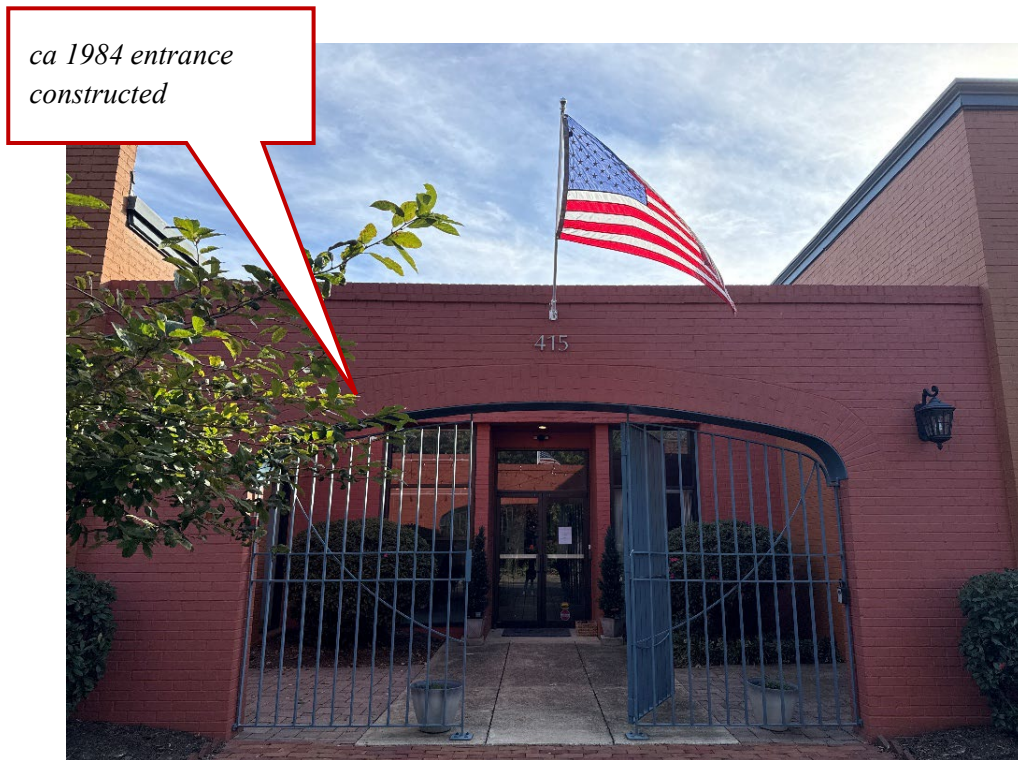
Figure 18: Detail of Front Entrance Arch – West Elevation View to the East
