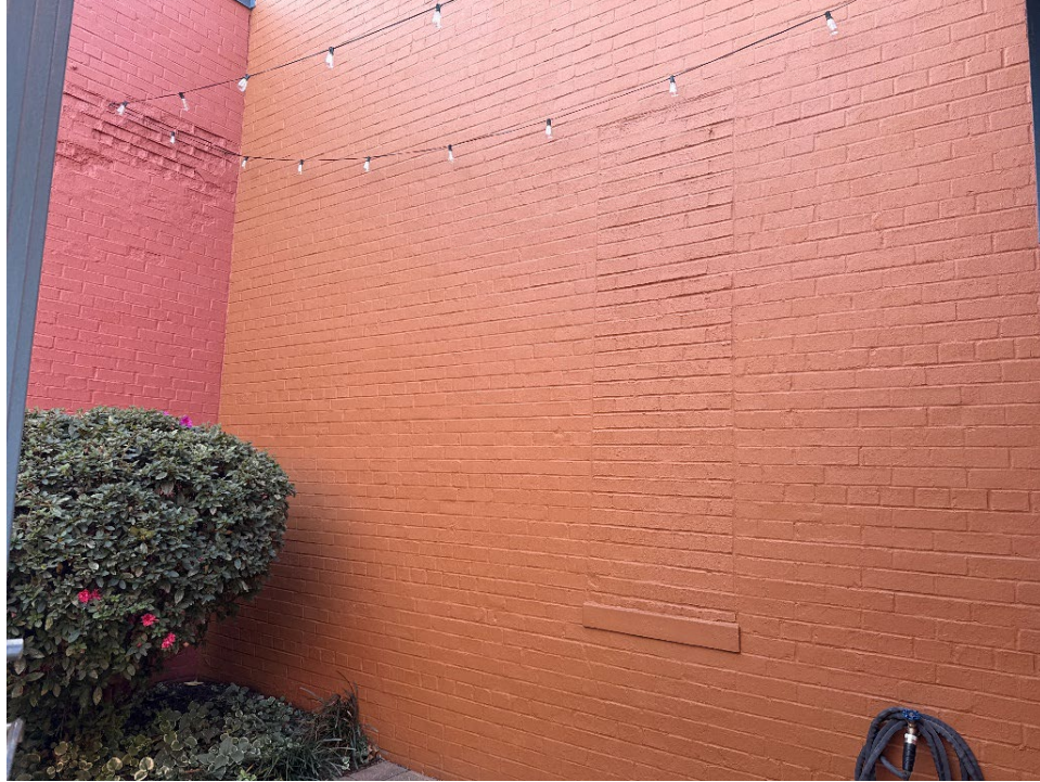
Figure 15: Detail of post-1950s section – North Elevation View to the Southeast
