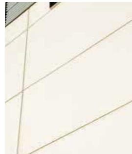
Siding - engineered stone panel (4'x8' nominal) rain screen, matte finish with reveals.
