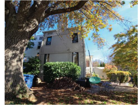
West facade @ Royal Street
