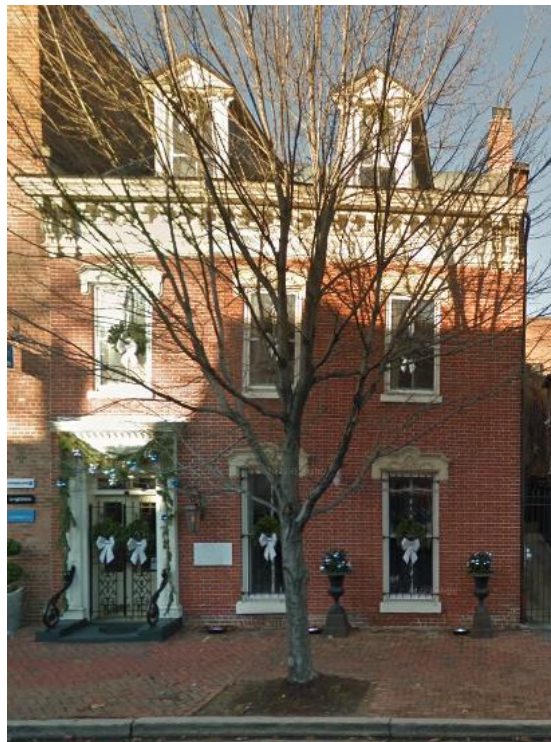
Photo 1: Existing facade of 111 S. Columbus St.
