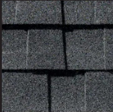
^ ARCHITECTURAL GRADE ASPHALT 20TH - 21ST CENTURY
