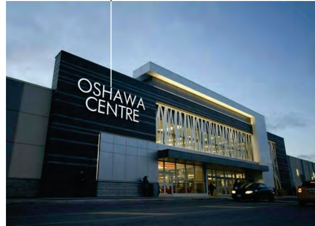
Face Illuminated Channel Letters Mounted to metal wall panels
