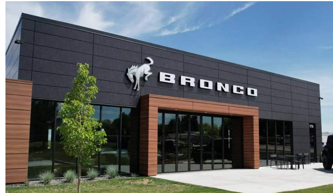
METAL PANELS AT HYPHEN: ALUMINUM PANELS BY MANUFACTURER PURE+FREEDOM - FINISH "BROOKLYN STEEL," WHICH IS A CHARCOAL GRAY WITH FAUX-PATINATION. APPLICATION SHOWN: BRONCO DEALERSHIP. KENDALL, FLORIDA.
