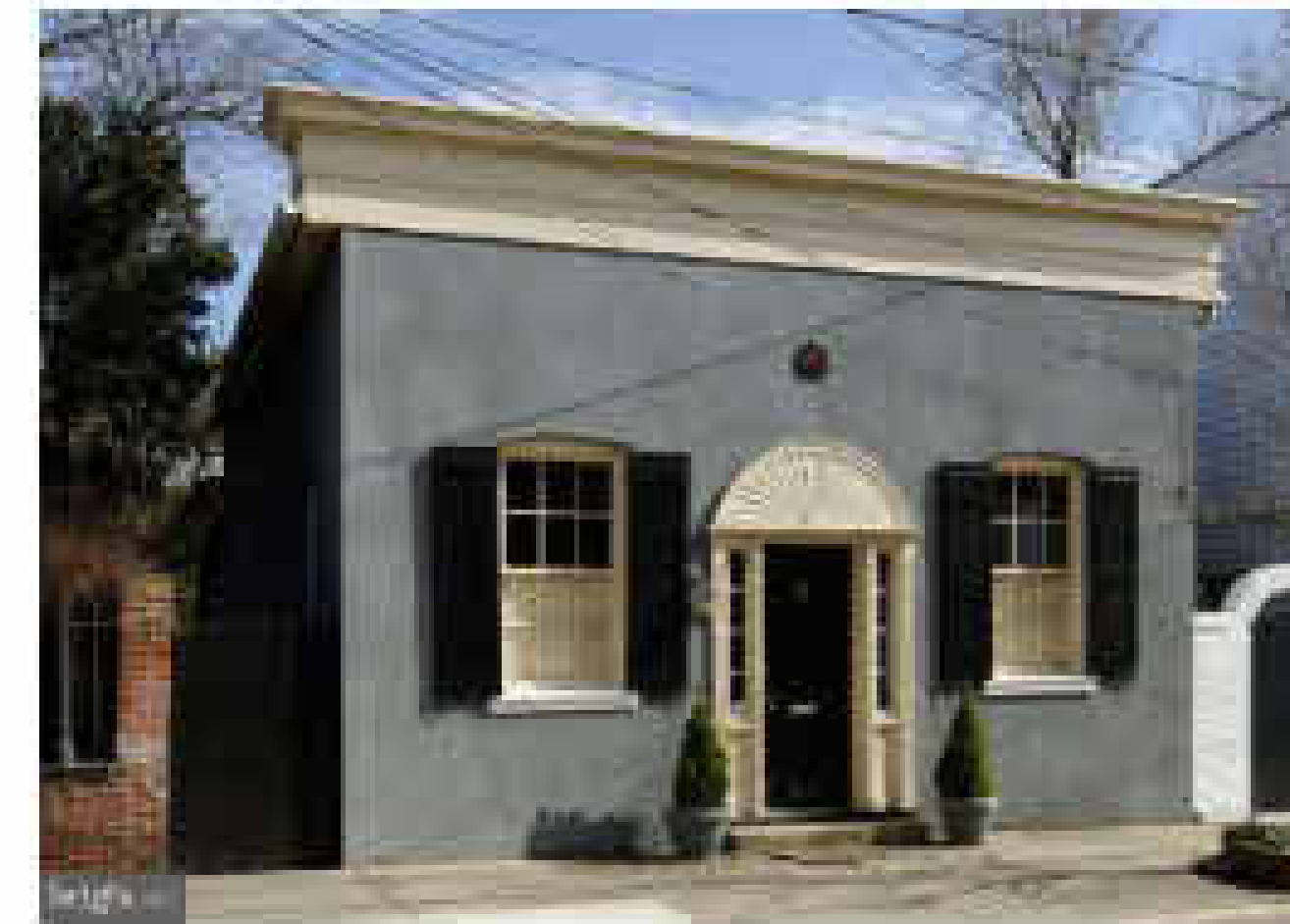
VIEW OF WEST ELEVATION AT 424 S LEE ST
