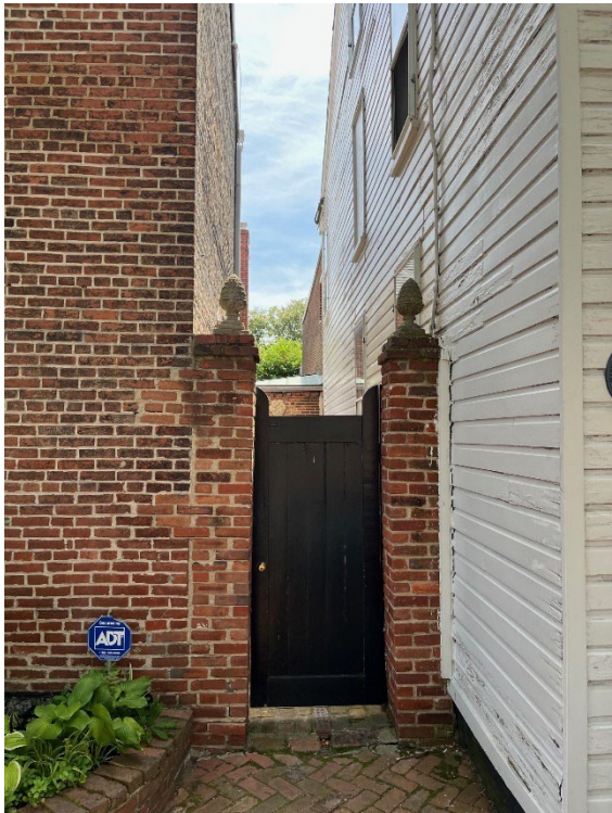
Figure 3: North side of house visibility
