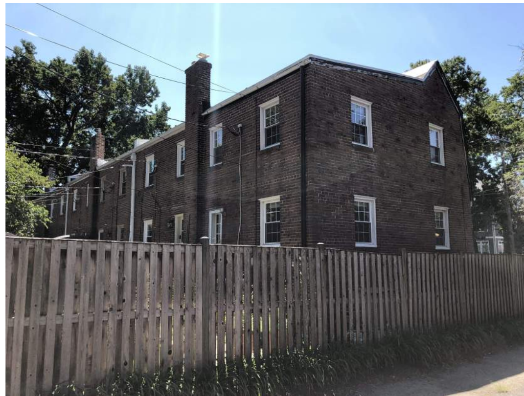
4. 1403 TO 1411 MT. VERNON AVE. REAR FACADES
