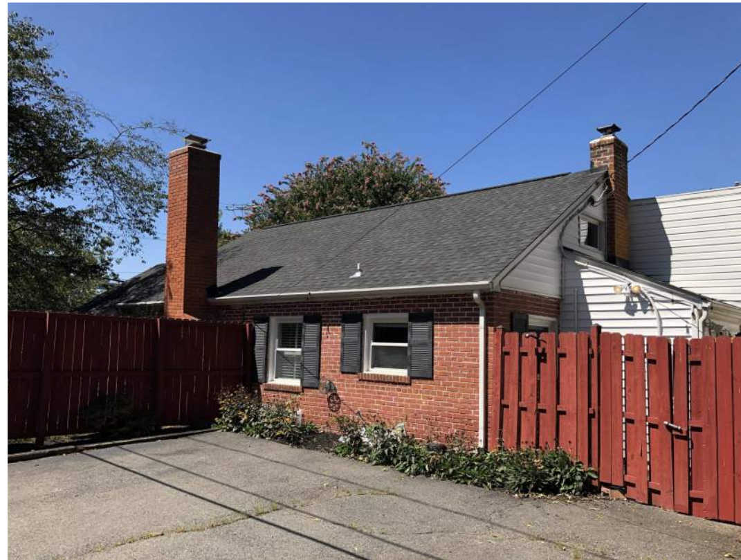
2. 1413 MT. VERNON AVE SIDE AND REAR FACADE
