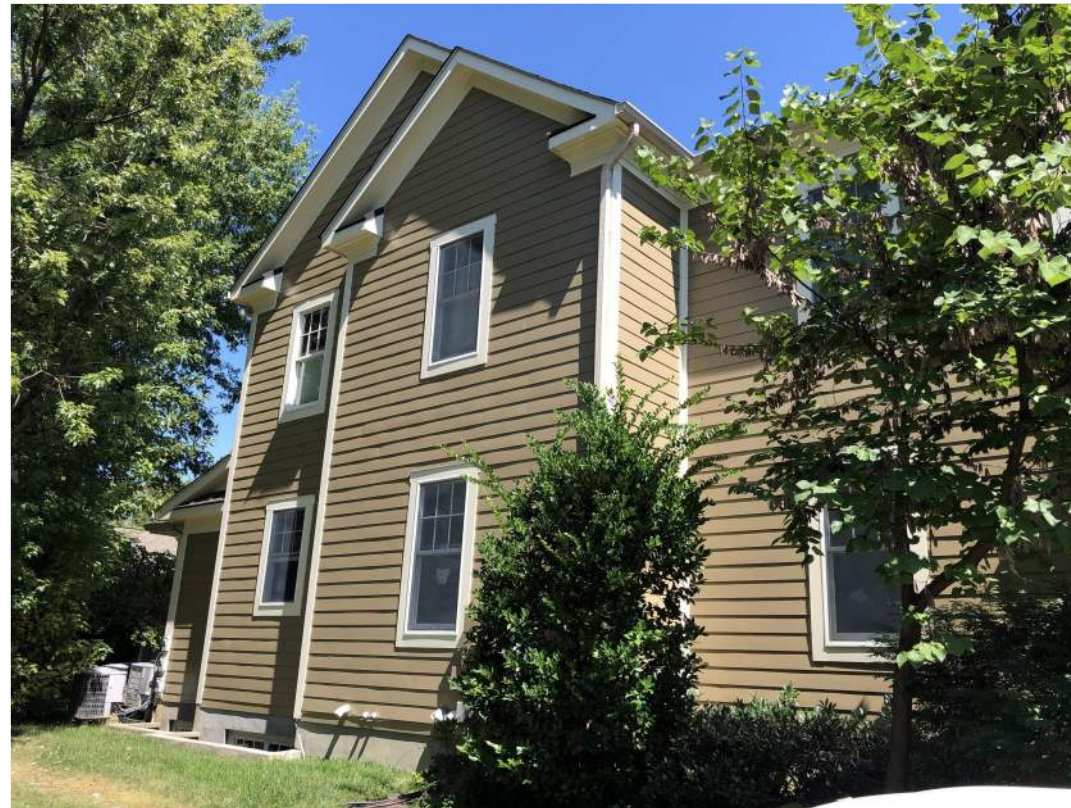
4. 408 E. ALEXANDRIA AVE. WEST SIDE YARD
