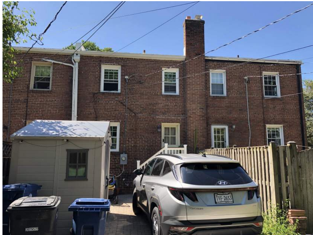
3. REAR FACADES AND YARDS OF 1407 - 1411
