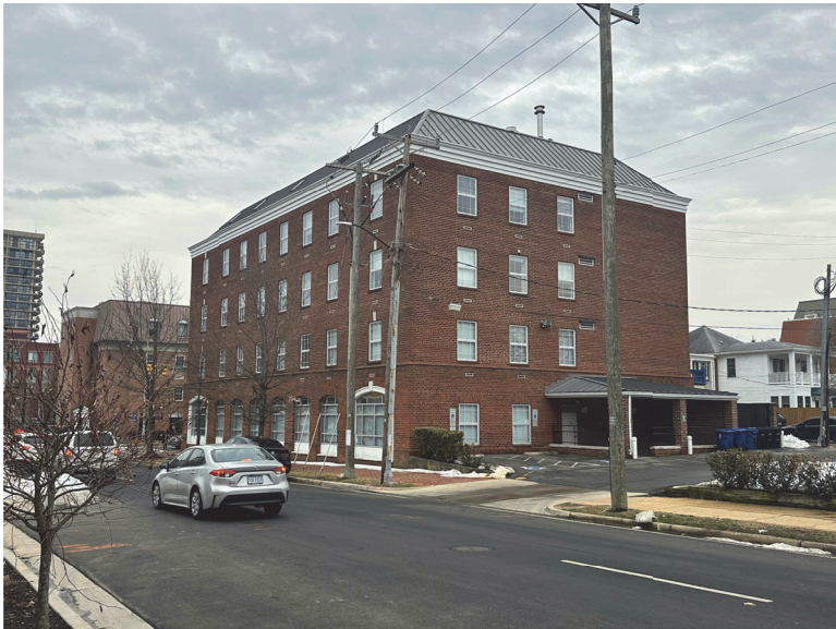
NW CORNER - MADISON ST AND PUBLIC ALLEY
