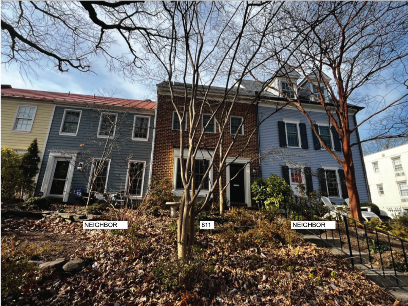
EXISTING FRONT ELEVATION - STREET VIEW 811 SOUTH COLUMBUS STREET
