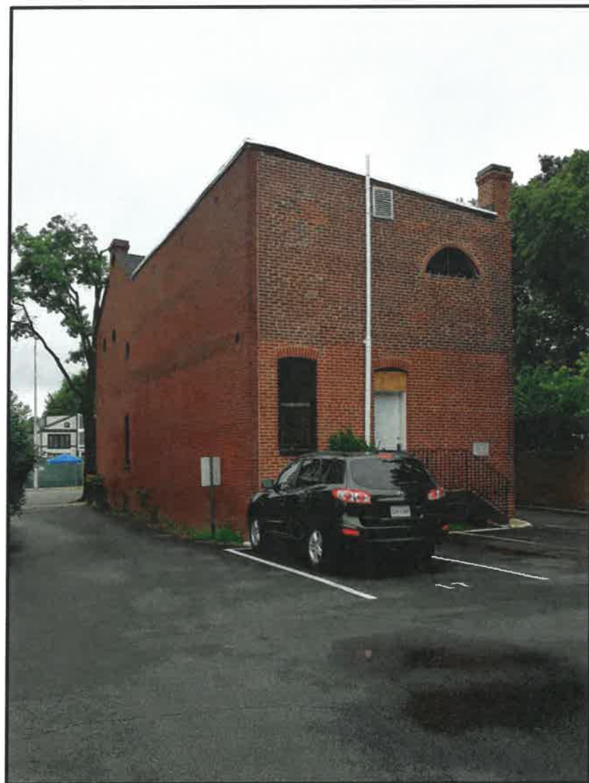
1 VIEW FROM SOUTH-WEST CORNER A03 SCALE: N/A
