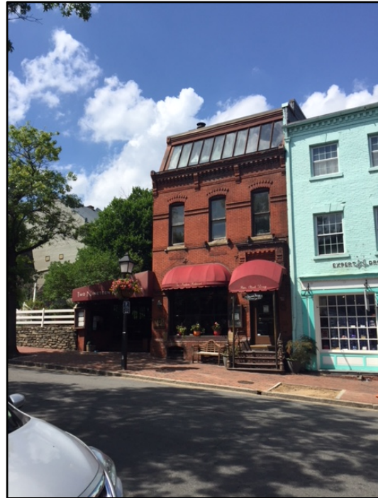
Figure 1. Front elevation, 219 King Street.
