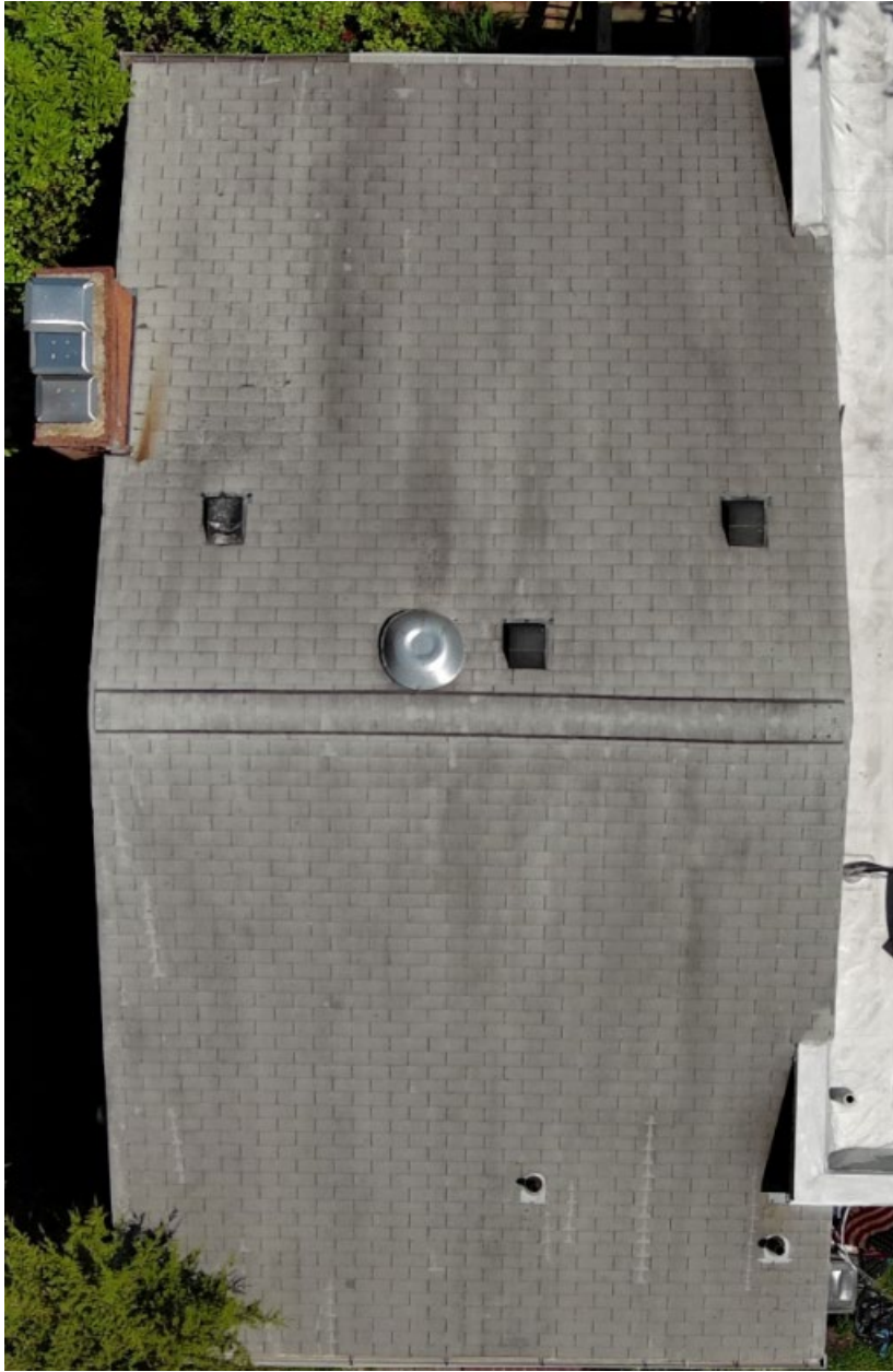
Full Scope of Roof
