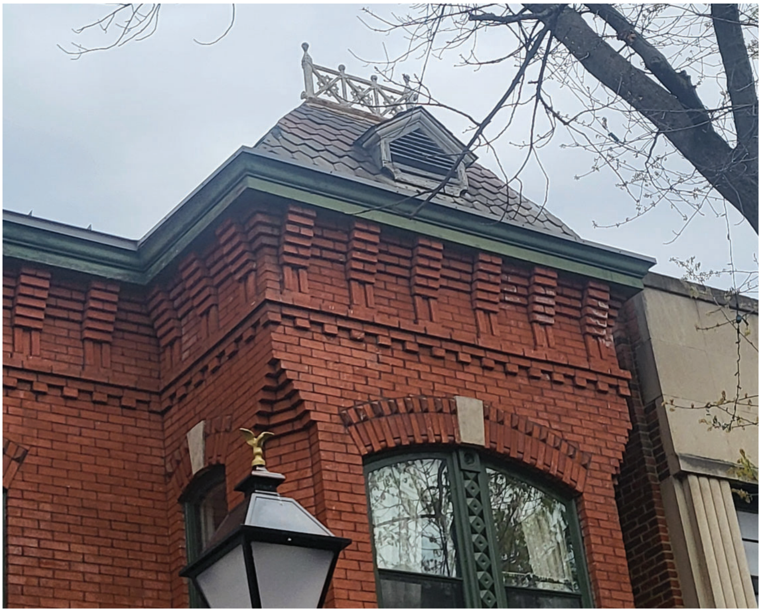
Roof element at 913 King Street
