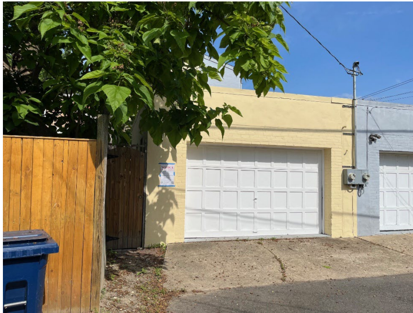
Figure 1: Garage behind 308 N. Columbus
