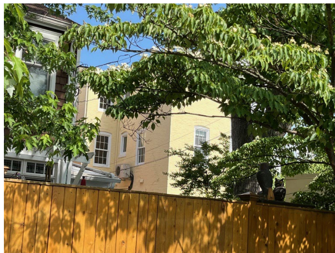
Figure 4: View of north elevation from public alley
