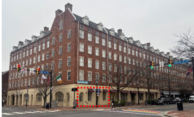
Photo 1: Existing conditions at 400 King St.
