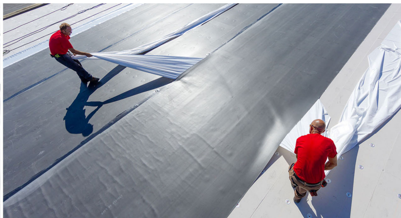
Firestone Fullforce EPDM SA Installation Photos
