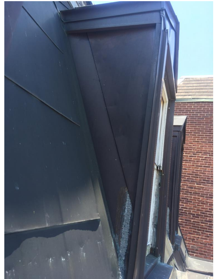
Copper roof and dormer cladding on the ca 1905 north dormers of the South Block to remain
