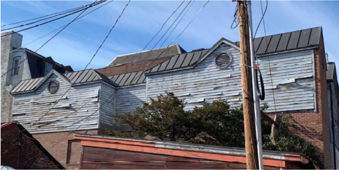
Figure 7: East elevation of 1985 addition
