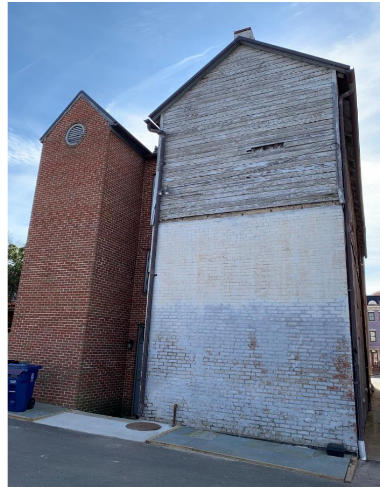
North Elevation: 1812 North Block, 1905 3 rd floor & 1985 Addition Photo: Gretchen Bulova 2021
