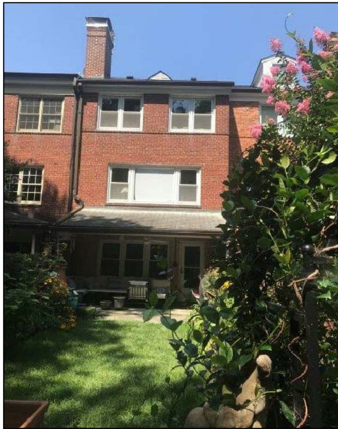
REAR EAST ELEVATION 820 SOUTH LEE STREET
