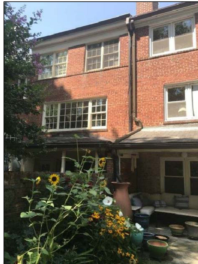
REAR EAST ELEVATION 822 SOUTH LEE STREET
