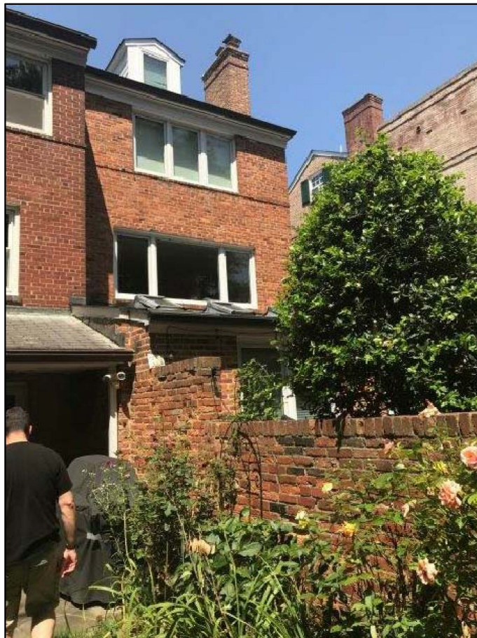
REAR EAST ELEVATION 818 SOUTH LEE STREET
