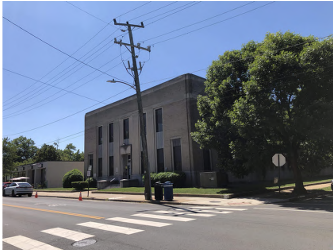
3. SOUTHWEST CORNER OF MT. VERNON AVE. & E. ALEXANDRIA AVE.
