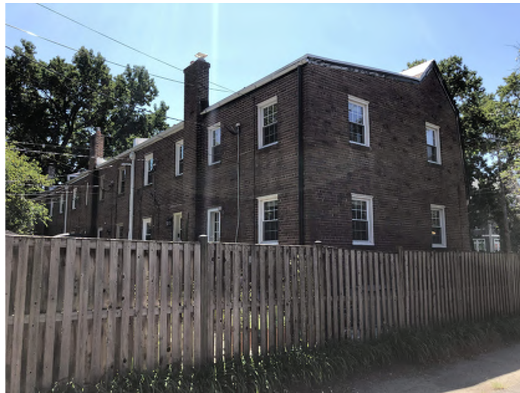
4. 1403 TO 1411 MT. VERNON AVE. REAR FACADES
