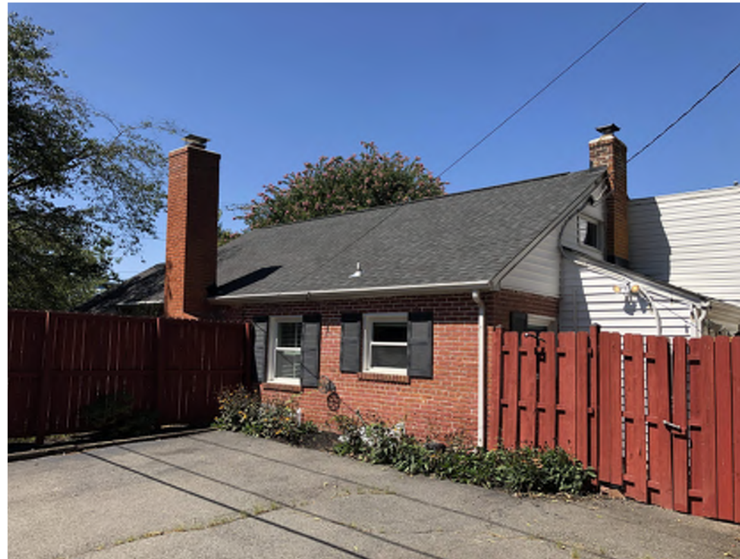
2. 1413 MT. VERNON AVE SIDE AND REAR FACADE
