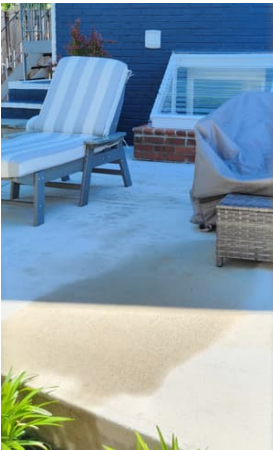
Dry floodproofing, protection around basement window.
