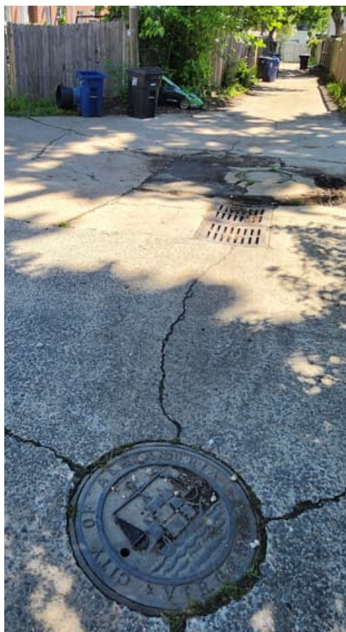
Storm drain and sanitary structures adjacent to houses.
