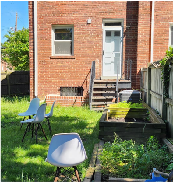
Brick wall/steps installed around basement entrance to block surface runoff.
