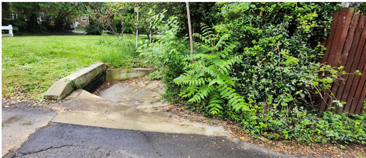
Opening of Hooffs Run Culvert adjacent to backyard of a structure.
