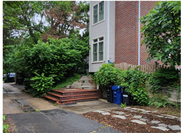
Lower basement entrance protected with wall/steps adjacent to storm drain inlet.
