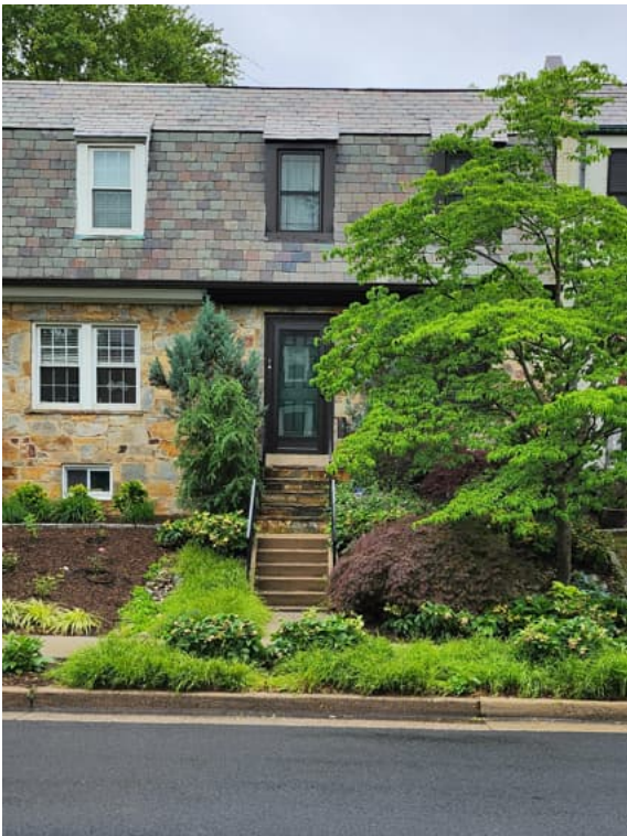
First floor and basement windows of building elevated above ground surface.
