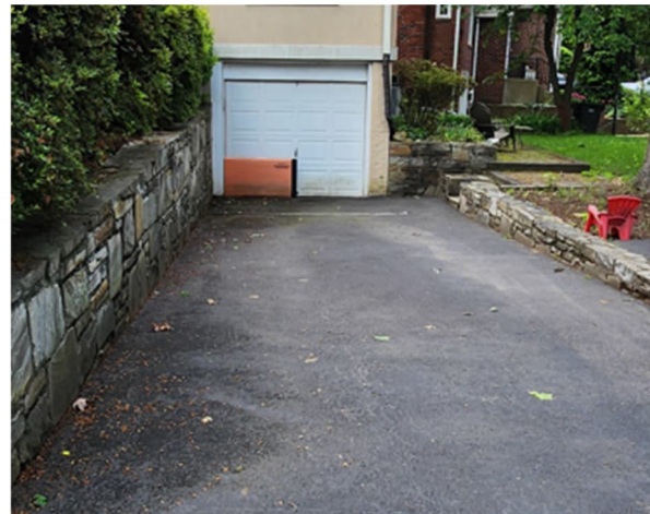
Dry floodproofing, floodwall at garage entrance.
