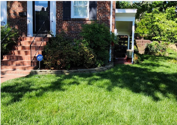
Elevated front entrance and lower basement entrance protected with wall/steps.
