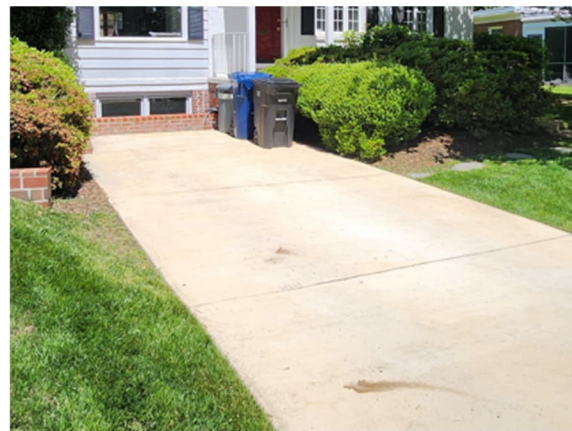
Re-graded driveway with barrier.
