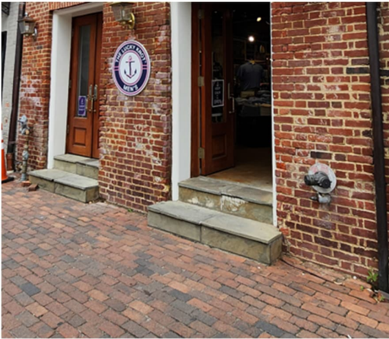
Elevated first floor entrance.
