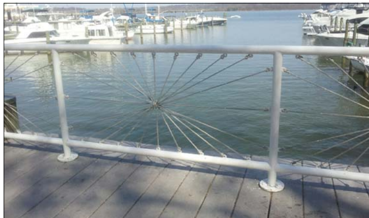
PHOTOGRAPH OF EXISTING RAILING AT MARINA
