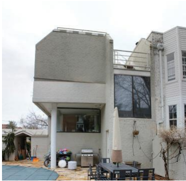
East facade @ Alley
