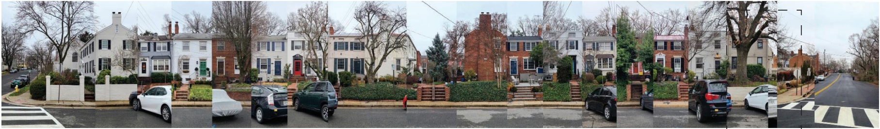
Existing Streetscape @ Royal Street
