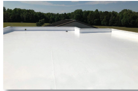
Low slope roof (fluid applied OR TPO (Thermoplastic Polyolefin) membrane color - white
