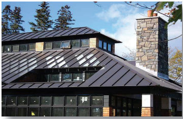
Metal roof examples (standing seam metal @ ±21" o.c.)
