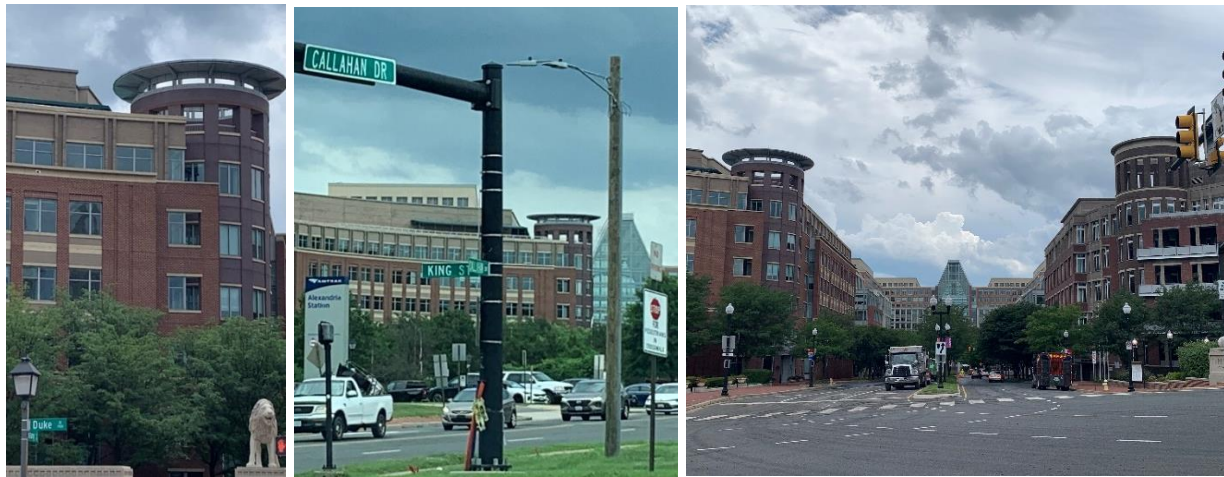
Figure 1: Views of the Existing Tower Architecture
