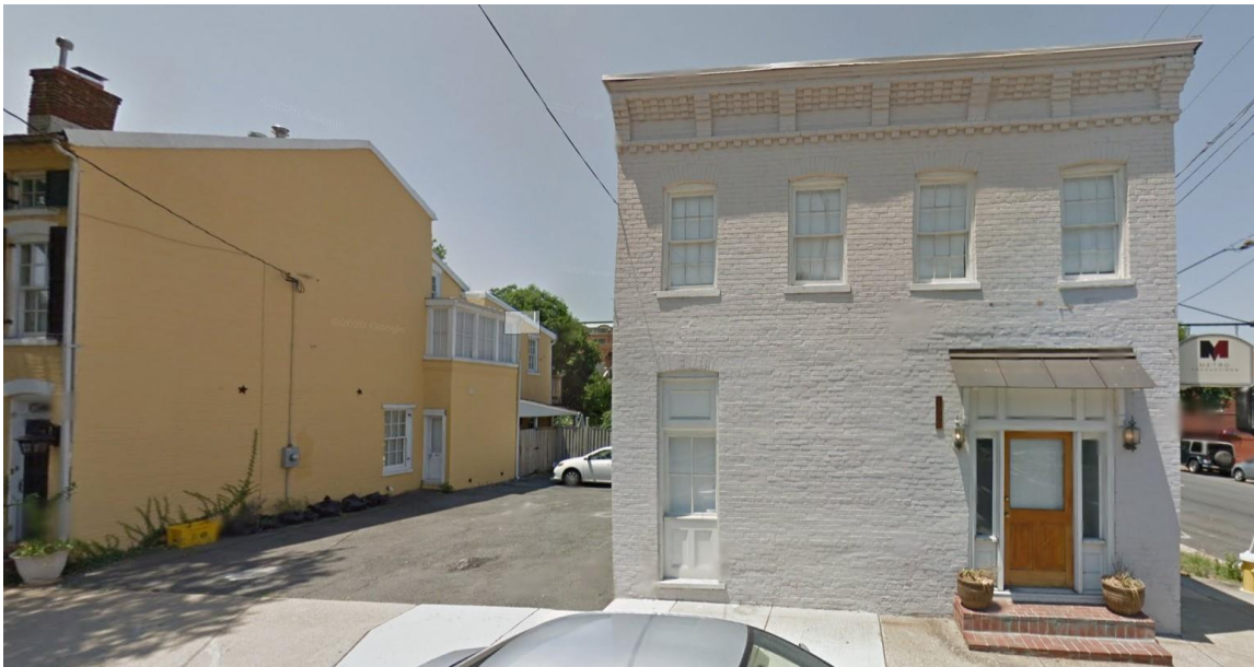
Existing Parking Lot
