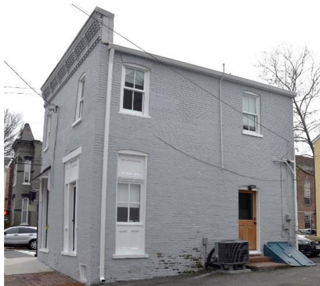
Figure 3: West elevation showing bulkhead and height of parapet
