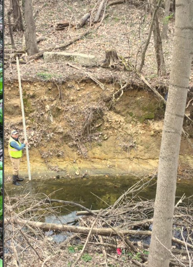
Exposed sanitary sewer
