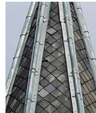
3 DIAMOND SHAPE SLATE ROOF TILE TYPE B
