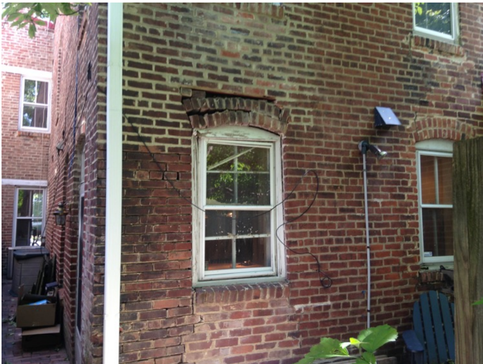
REAR WALL (SOUTH ELEVATION)
