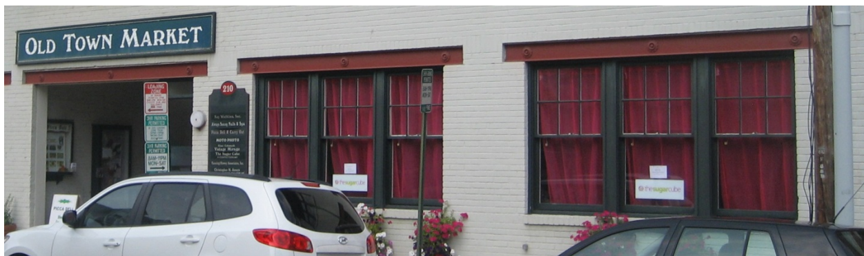
Figure 6: Steel C-channel lintels above triple windows at 210 N. Lee Street.
