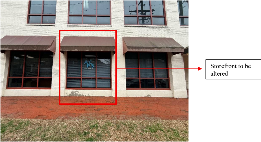
Figure 3 - Existing storefront composition
