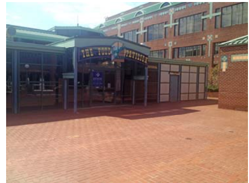
Rear deck on northern portion of site proposed for outdoor dining
