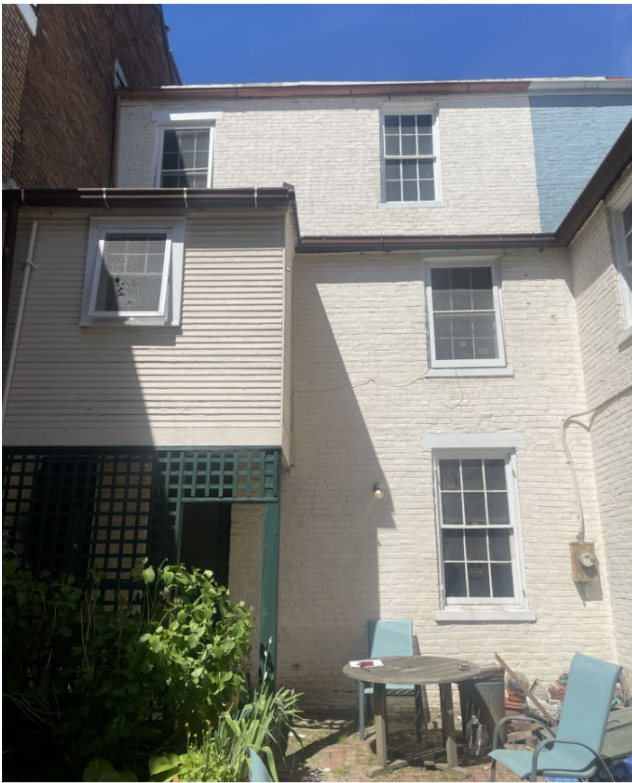
Figures 2&3: Frame area to left to be demolished; two-story brick portions in both images to be rebuilt
