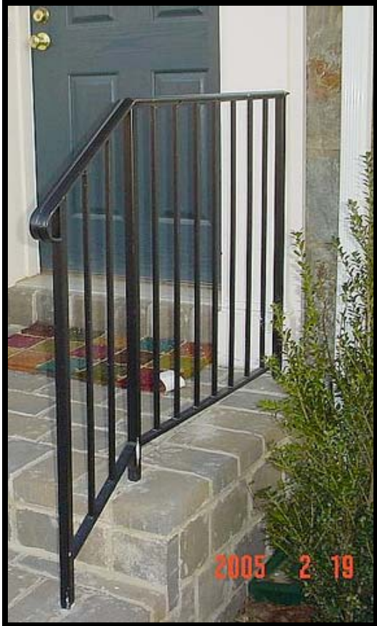
Front Entrance Porch Railing Detail
