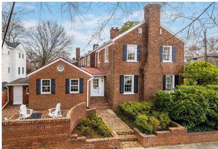
Photo 1: Existing east garden wall.
