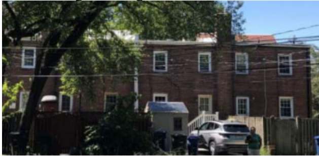
Rear of townhouses on Mount Vernon Avenue
