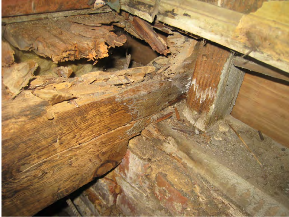
Figure 9 - Condition of floor and framing in existing rear "el" addition
