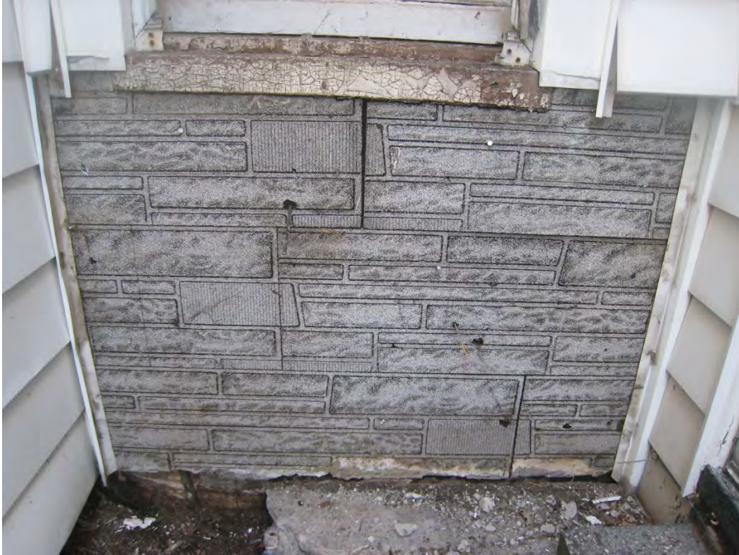
Figure 3 – Asphalt siding on east elevation of main house block visible after removal of aluminum siding
