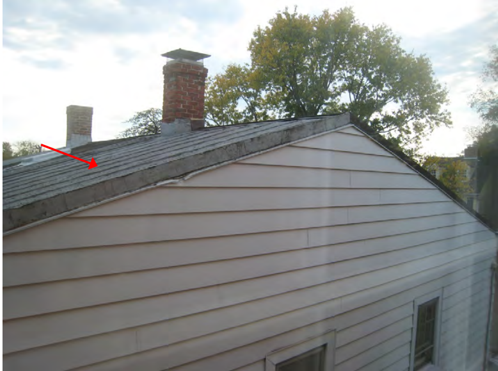
Figure 7 – View of rear roof slope of main house block
