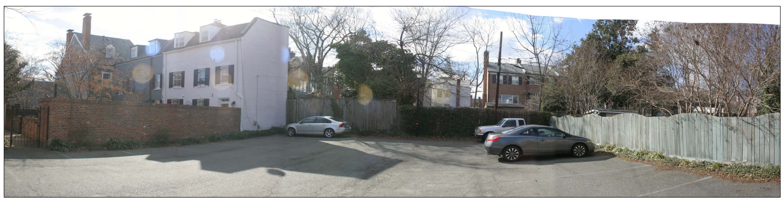
9 VIEW OF THE REAR OF 418 SOUTH PITT STREET LOOKING WEST A5 SCALE: 1" = 10'-0"
