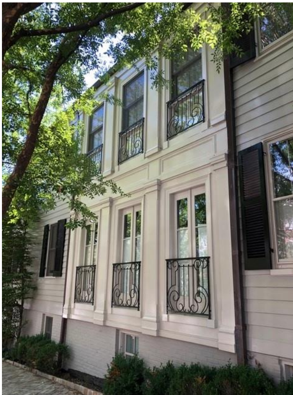
Figure 6: 300 South Lee Street
