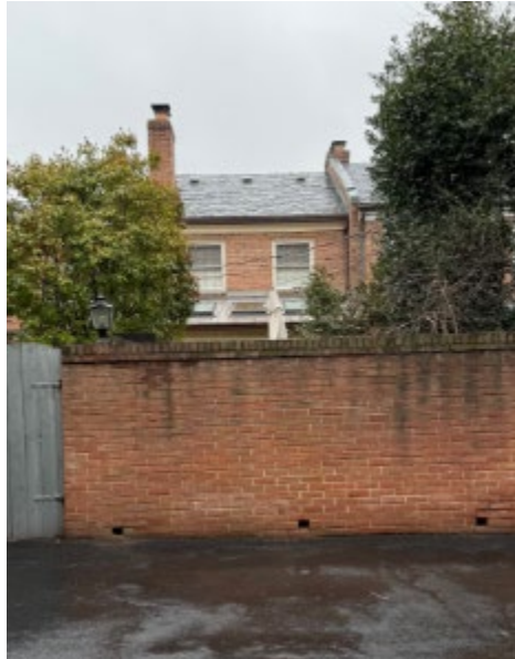
Photo 1: View of rear (east) elevation.
