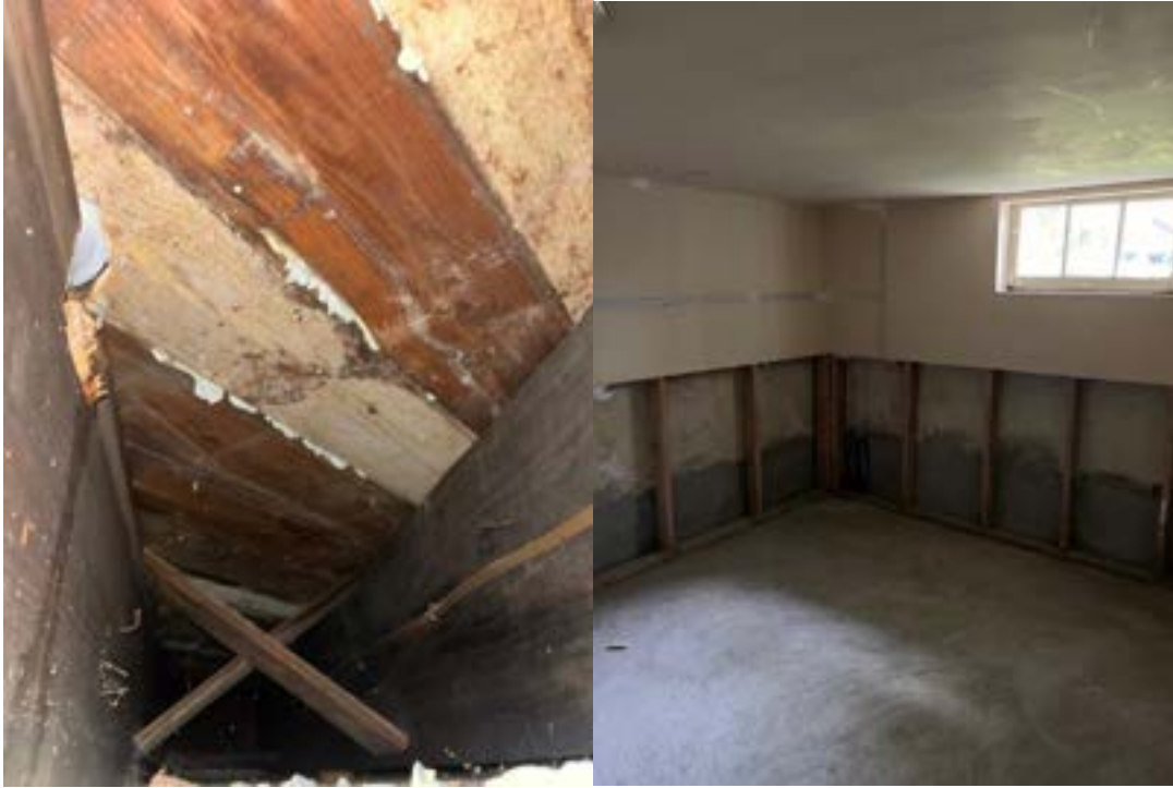
Photo #1: JOIST PHOTOS FROM BASEMENT
